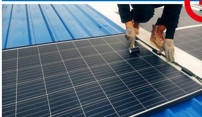
Quick-bonding粘贴安装
